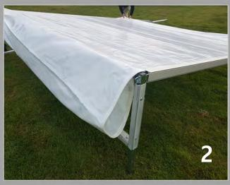
**Step 7:** Now feed both sides of the roof panel (the keder beads) into 'F' Main Long Roof Beams at the same time and same speed. Photo 3 and 4 show the roof sheet sliding down the channel of the roof beams, now your roof will be glossy side up and installed correctly. Make sure the roof sheet is pulled down evenly to prevent jamming and all of the way to the bottom.
