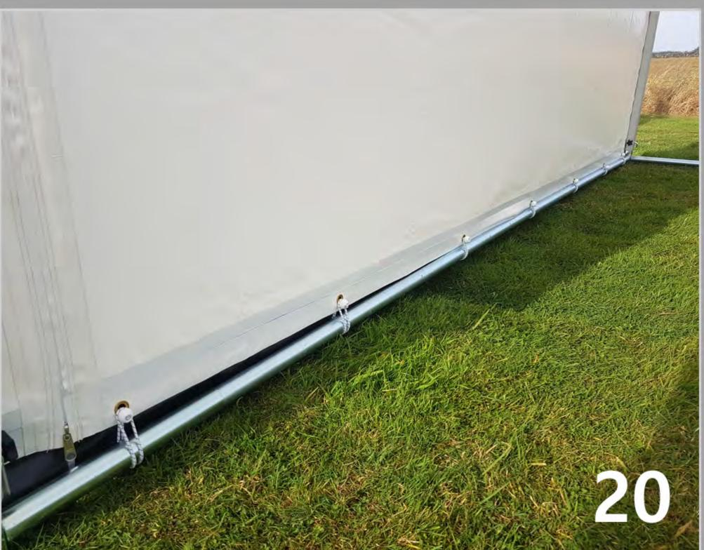
**Step 15:** Tension the floor rail by sliding the cap and extending the Floor Rail 'K' so it becomes longer. At the bottom edge of the all of the walls are elastics which are pulled around the Floor Rail 'K' and back onto themselves. In the above Photo 20 you can see the elastic being used.
