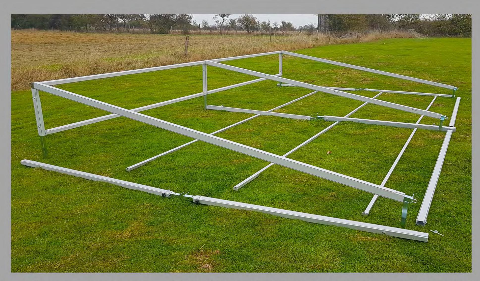
**Step 4:** Drop Components 'C' Roof Spreader Bars into the brackets located on the sides of 'F' Main Long Roof Beams.
