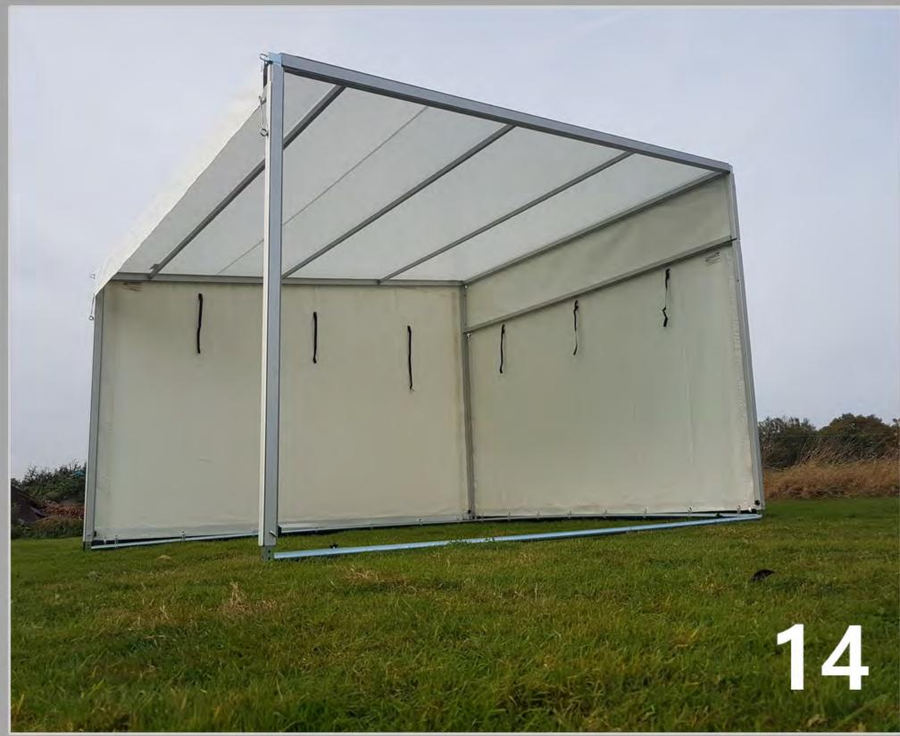
**Step 12:** At the back, slide the back walls into the lower outside groove on the Back Beam Top 'E' as shown in Photo 13. When slid all the way across, unzip both sides of the back walls and slide the bead into the groove on the leg.
