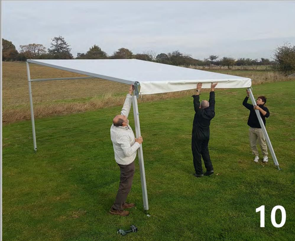
**Step 10:** Lift the back of the framework up and slot on the legs, making sure the nut eyes and feet are pointing outwards on all legs. Then, at the front of the awning, lift up the frame once again and slot on the legs, see Photo 10
